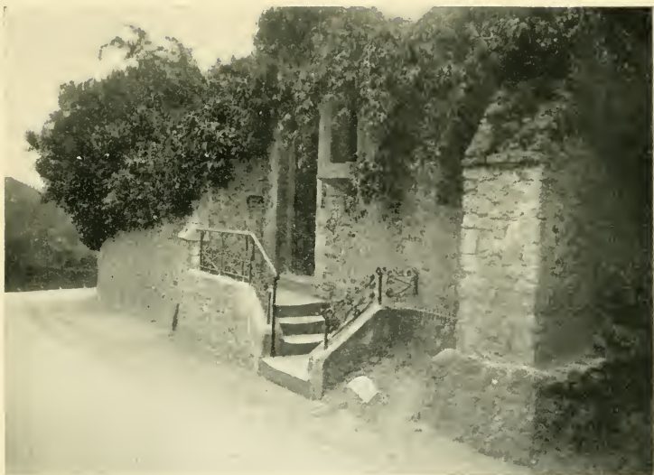
SIDE GATEWAY, DAVINGTON PRIORY.
